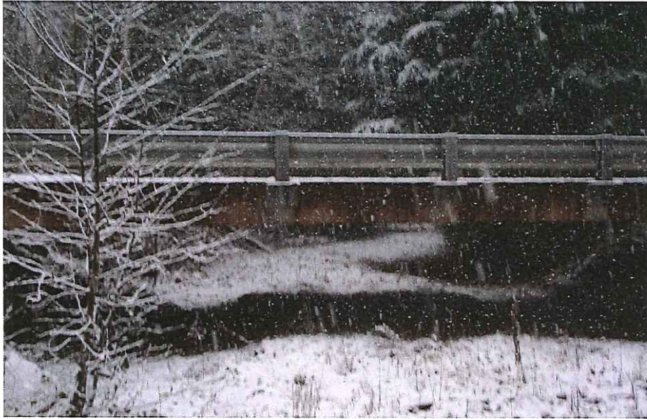
CK-2045 Crossing Upstream
