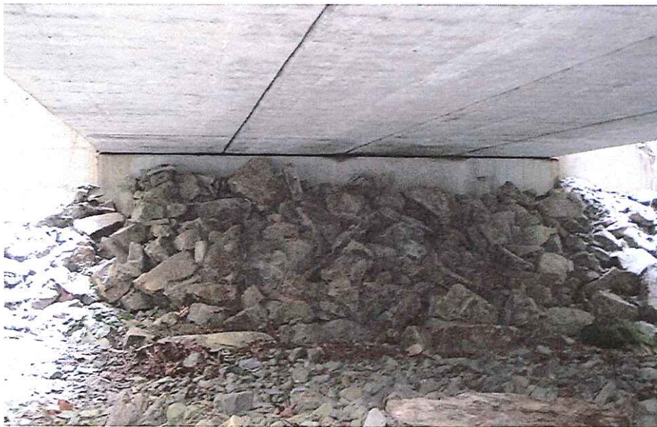
CK-2045 Abutment Right Bank
