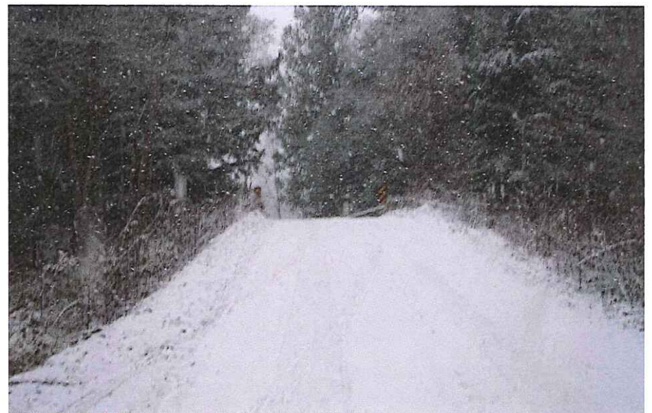
CK-2045 Approach Left Bank
