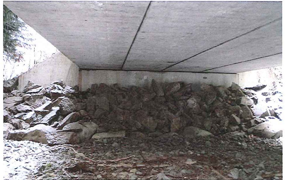
CK-2045 Abutment Left Bank
