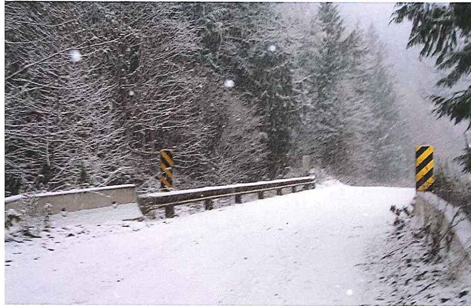
CK-2045 Approach Right Bank
